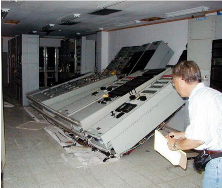
Photo: Overturned equipment in the 1985 Mexico earthquake.
