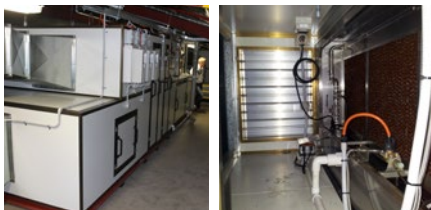
Solar desiccant TAC unit and evaporative cooler
