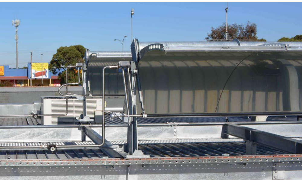
Configuration of simple desiccant cooling system
