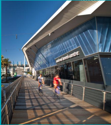
Image Courtesy of Watpac Construction
