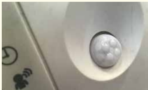
Figure 3: A PIR sensor used for energy saving on a Daikin split system indoor unit. Source: Dennis Kenworthy
