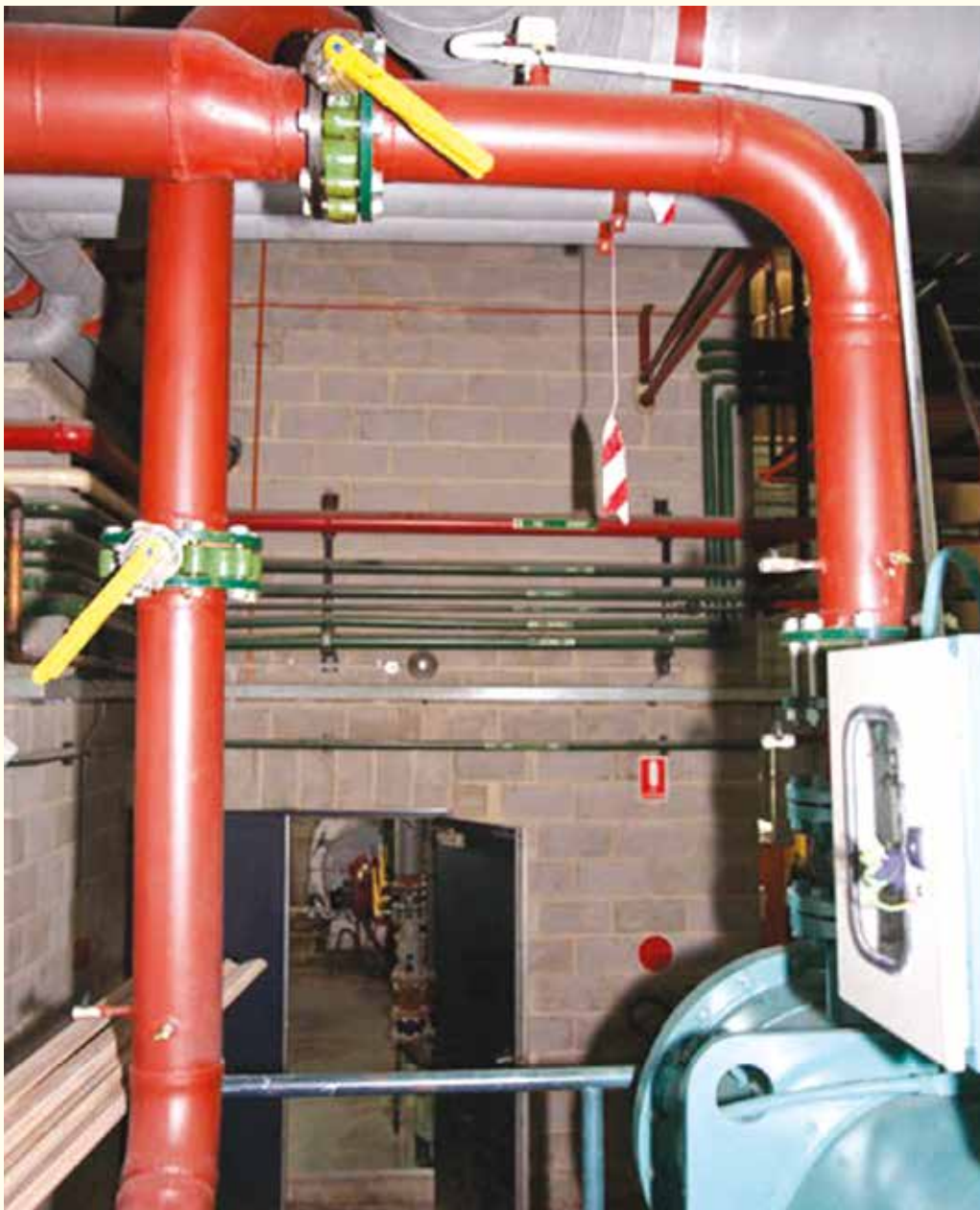
Throttled (choked) distribution system.
