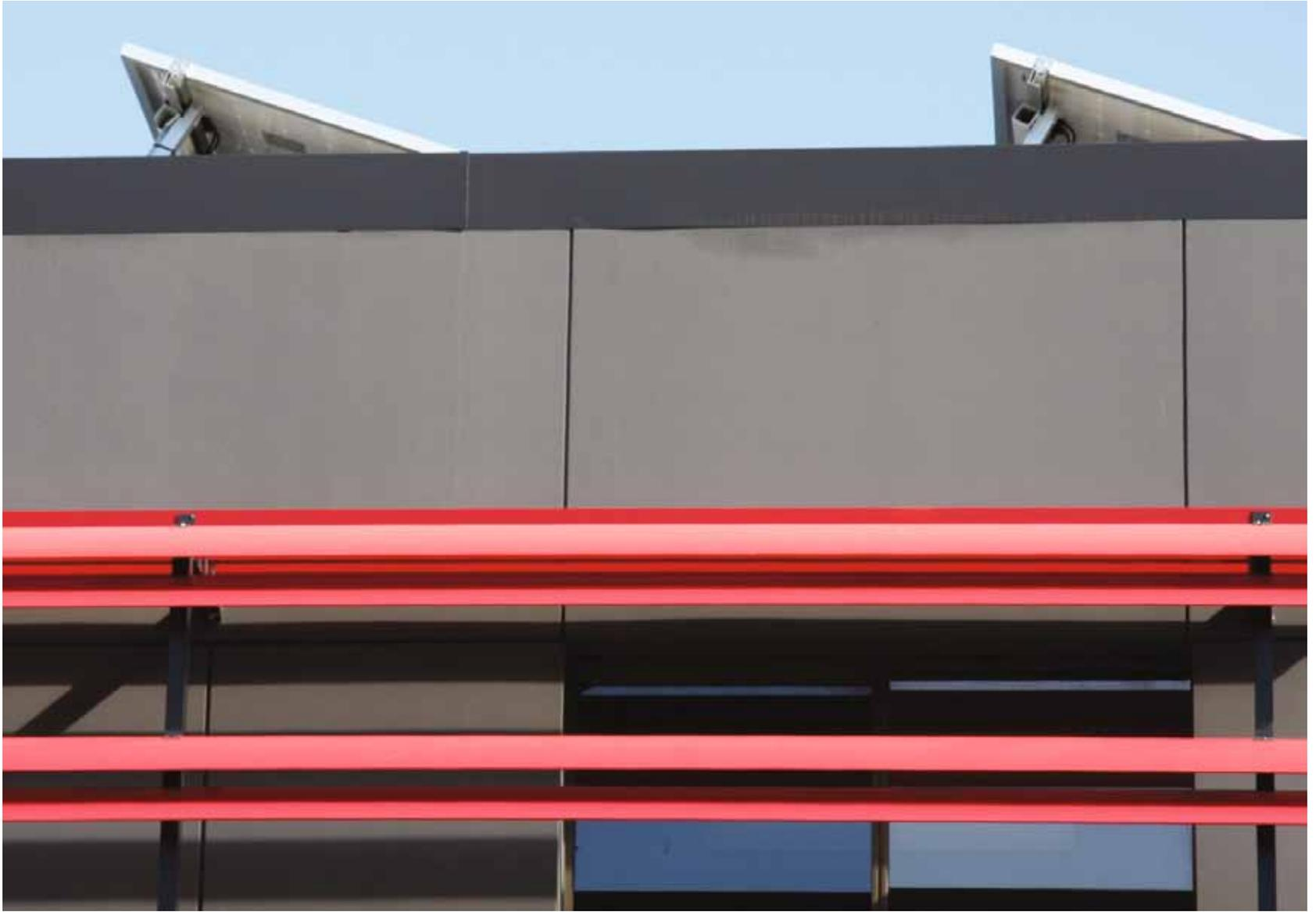
*As part of the retrofit, aluminium louvres were added to a number of windows to provide shading.*
