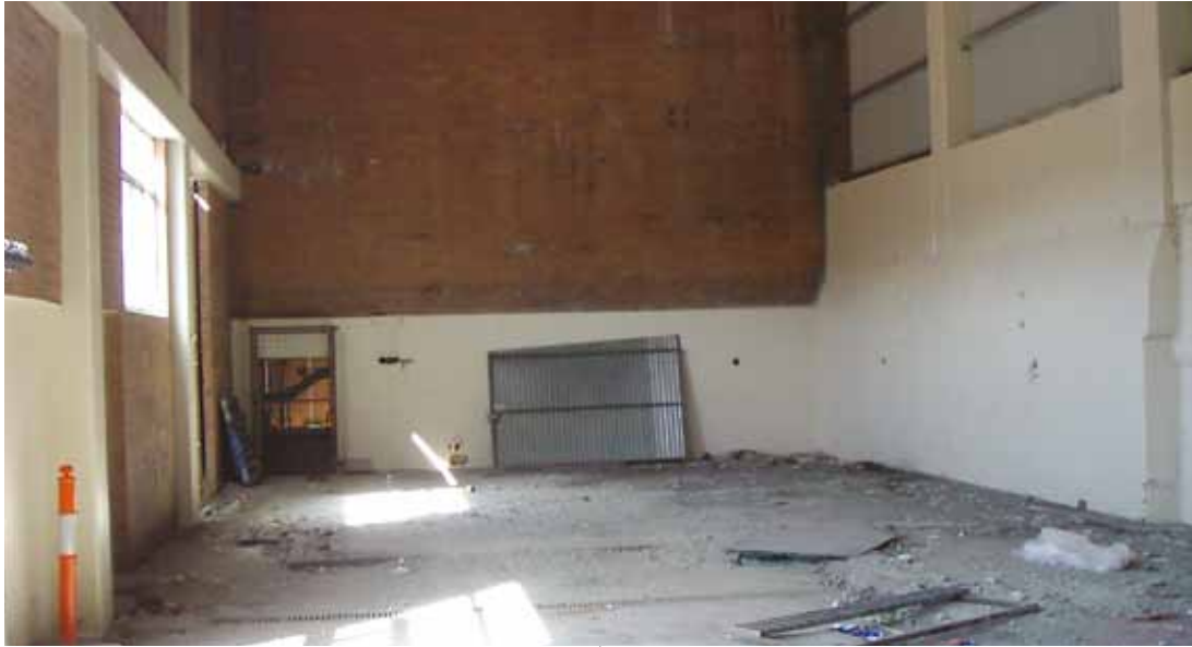
The plant room prior to the upgrade.
