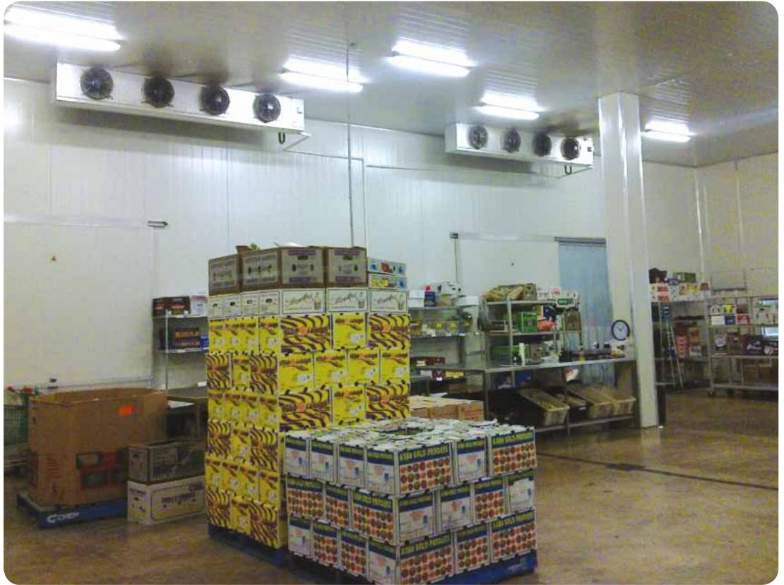
Two evaporators are utilised in the mango room.
