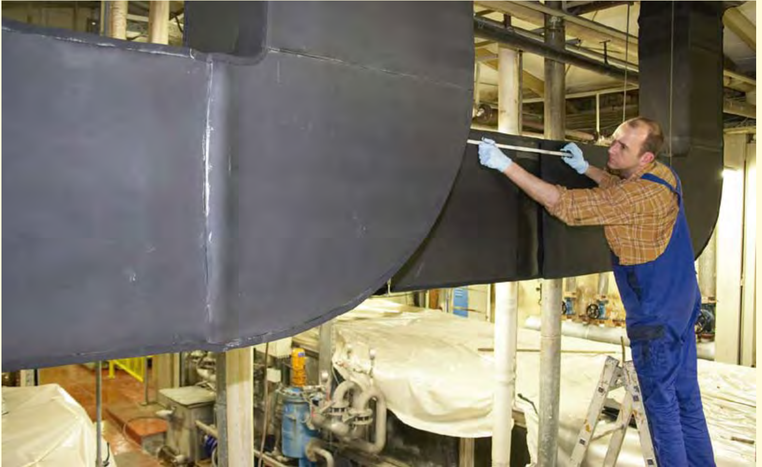
Duct being wrapped
