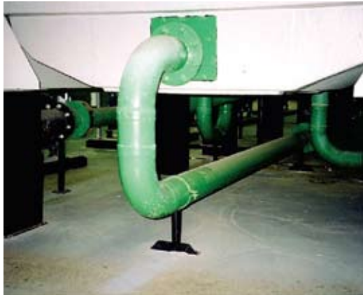
Fig 6. Balance line acts as a deadleg, impossible to drain.
