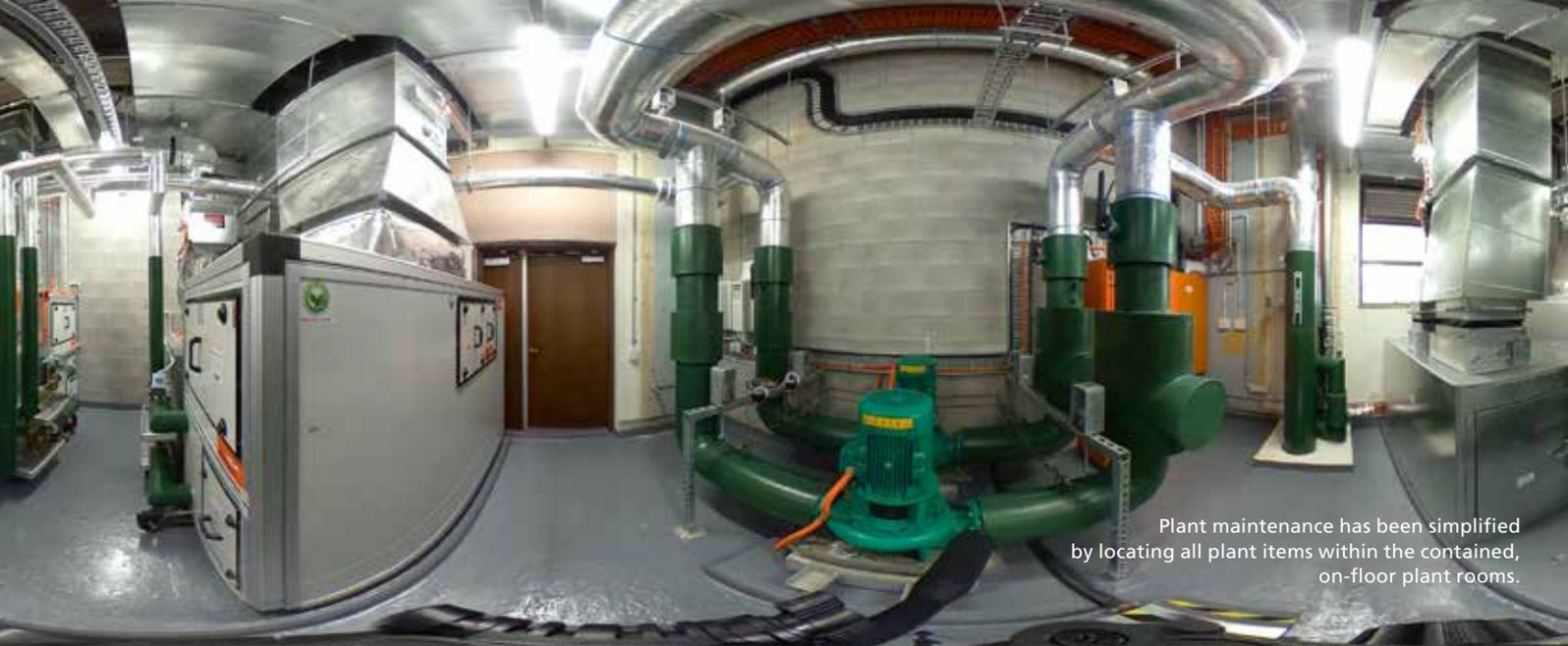
Plant maintenance has been simplified by locating all plant items within the contained, on-floor plant rooms.
