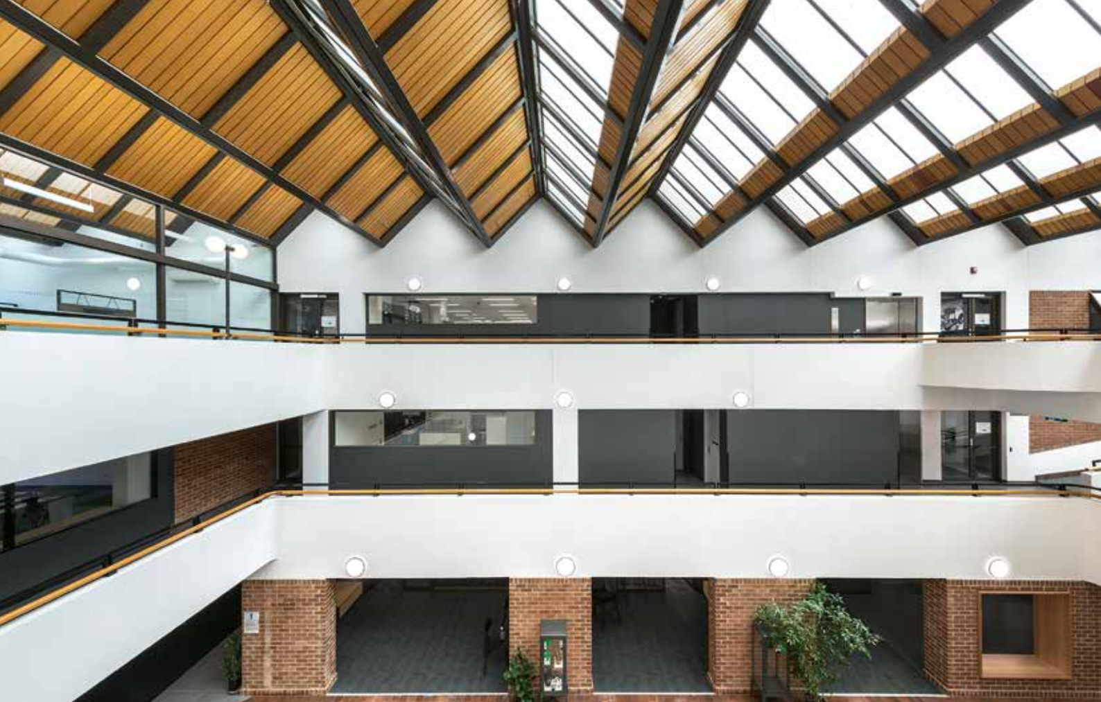
The building's main feature is its entrance atrium, with a full-height ceiling and skylight roof.
