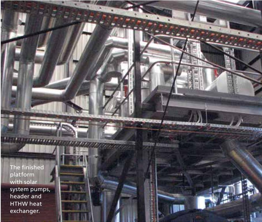
The finished platform with solar system pumps, header and HTHW heat exchanger.
