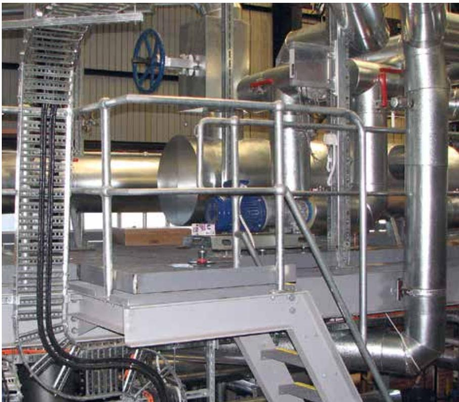
The solar heat exchanger and header system on the platform, during install.
