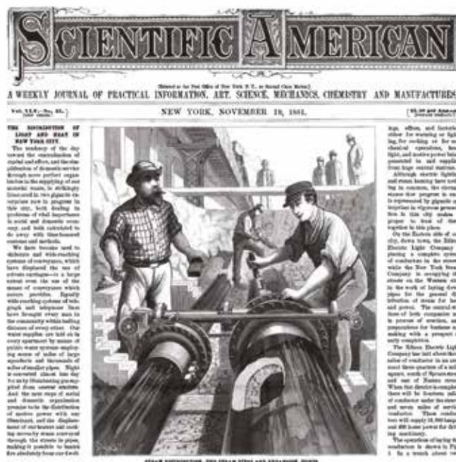
Figure 1: November 19, 1881 Scientific American magazine cover showing steam piping installation in New York City. Image courtesy of David Wade, RDA Engineering.
