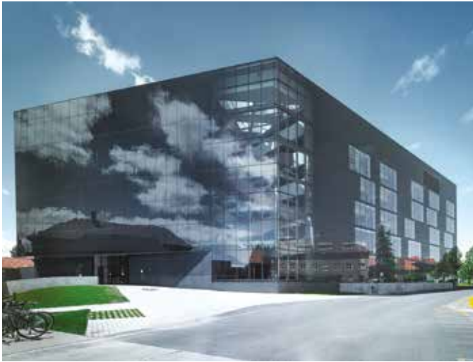
Figure 7: The building uses a combination of water and air based systems for energy efficiency. Photo: Mark Cramer
