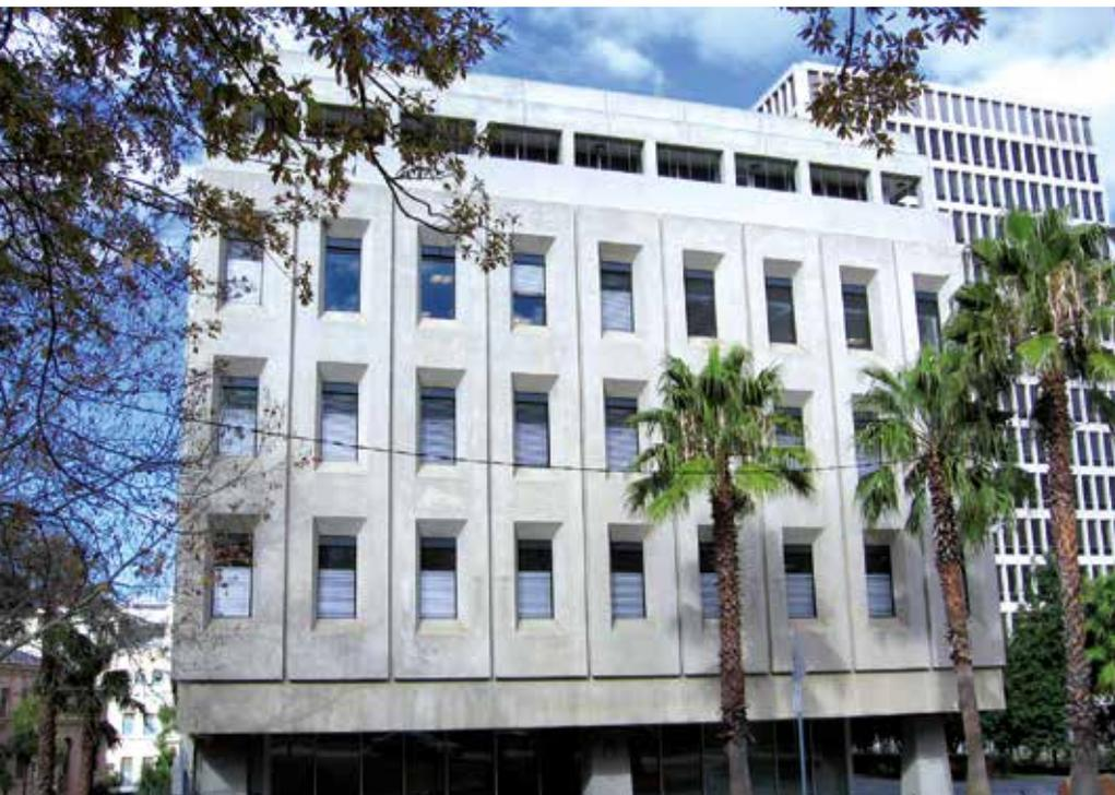
External automated blinds installed at Melbourne's 55 St Andrews Place control solar load. Image courtesy of Cundall.
