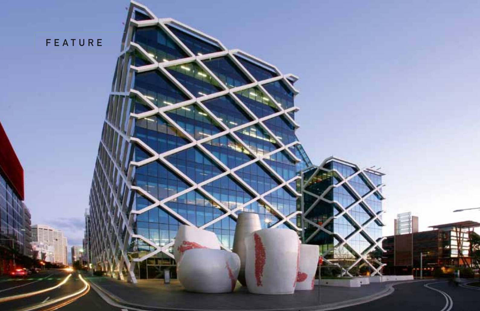
The building is wrapped in a diagonal grid of 3,000 tonnes of steel.
