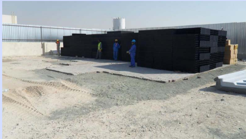
Comfort cooling using PVC fill without water
