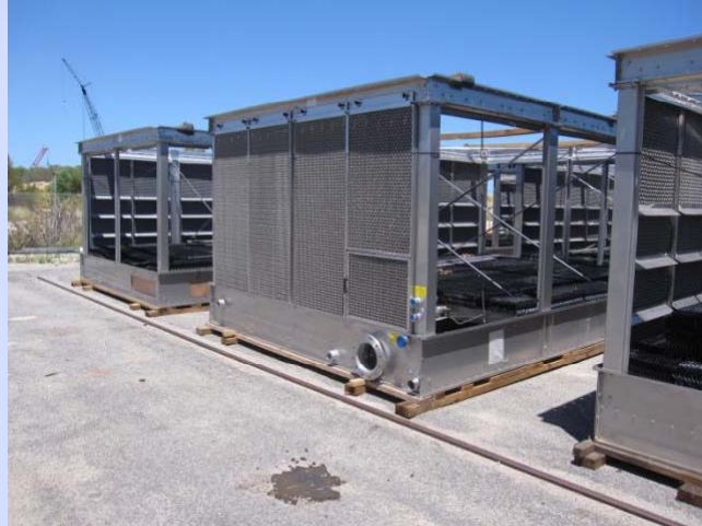
Efficient inlet louvers prevent splash out
