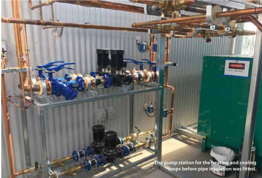
The pump station for the heating and cooling loops before pipe insulation was fitted.
