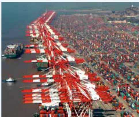
Port of Shanghai, China
