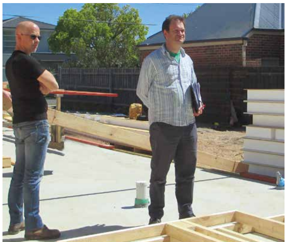
Habitech Systems' managing director Chris Barnett on site with senior architect Jon Pye.
