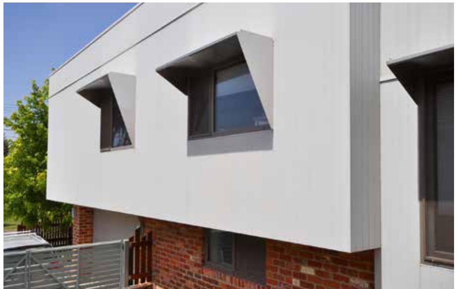
The trademarked modular shading system optimises shading to individual windows.
