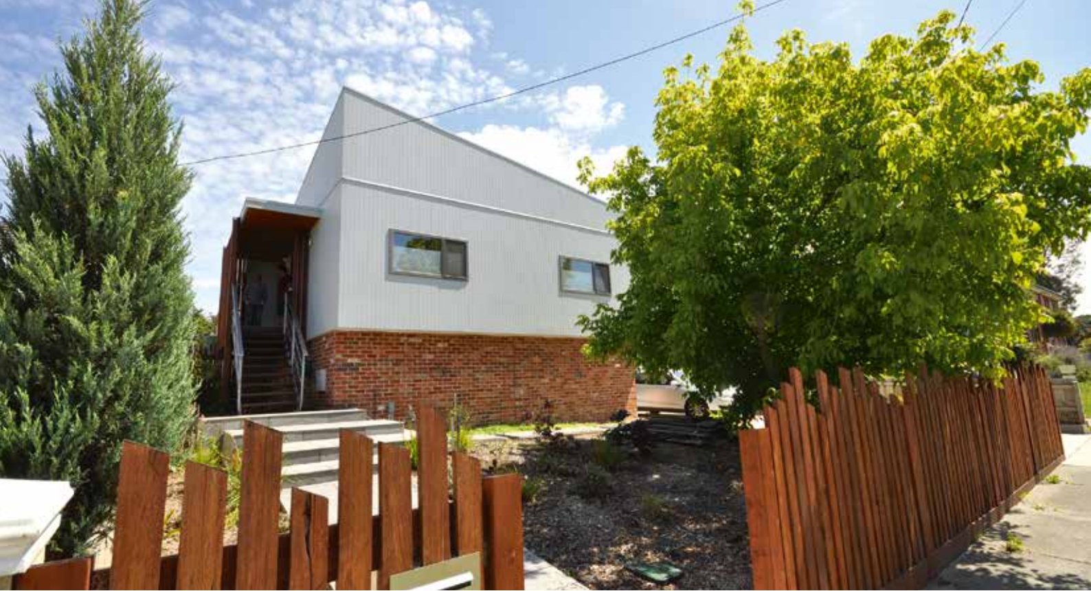
The street facade form was generated by the mounting of PV panels.
